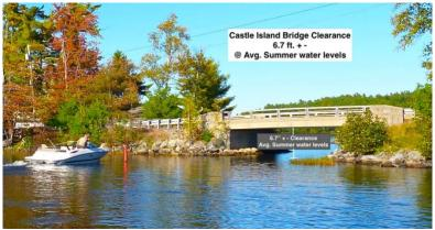
In the middle of the summer when Long Pond is at full pond (ie. water is just barely going over the spillway at the Wings Mill Dam) there is just 6.5' of vertical height clearance. With a heavy rain event and/or Spring melt, the water can easily come up 10-12" so obviously you're down to just 5.5' of clearance. And around Labor Day, you can plan on having at least 10-12" additional clearance, or around 7.5'. Obviously, these guidelines are just estimates due to the variables.
